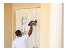
The Graco UltraMax Handhelds feature the new Graco FFLP Tips (Fine Finish Low Pressure) which dramatically reduces overspray while delivering a perfect finish.
